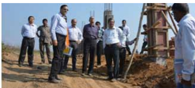
Dr. Ajay Kumar, IAS, Joint Secretary, DeitY and Dr. Ashwini Kumar Sharma, MD, NIELIT reviewing the progress at the construction site
